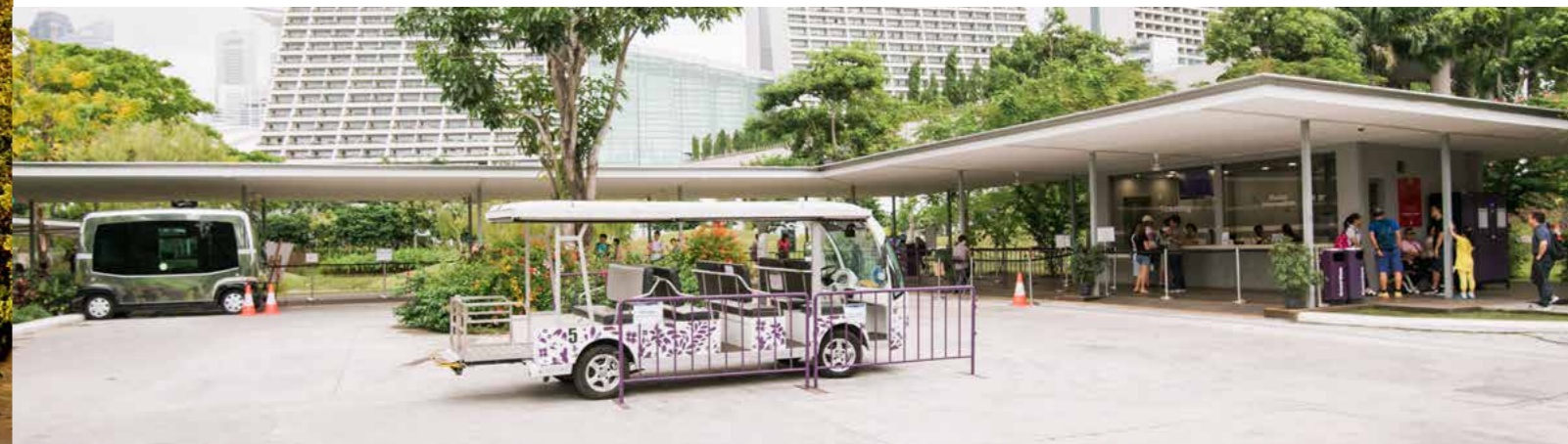
The new Bayfront Plaza, complete with Visitor Information and Ticketing counters, as well as a Shuttle Service stop
