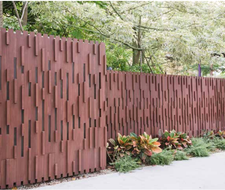
Feature wall along the new footpath connecting the Golden Garden to the Secret Life of Trees, built with materials sponsored by Samko Timber
